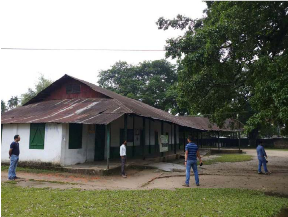
Figure 12. Hindi Vidyalaya near Makum railway junction. No cracks in the wall of the school or in the boundary wall are seen.
