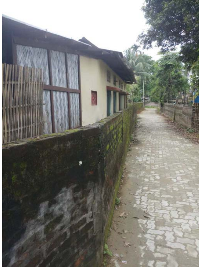
Figure 10. A long linear boundary wall in the Chabua town near the ITI building. No cracks in the boundary wall is seen.
